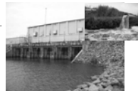
S-3 pumping station
